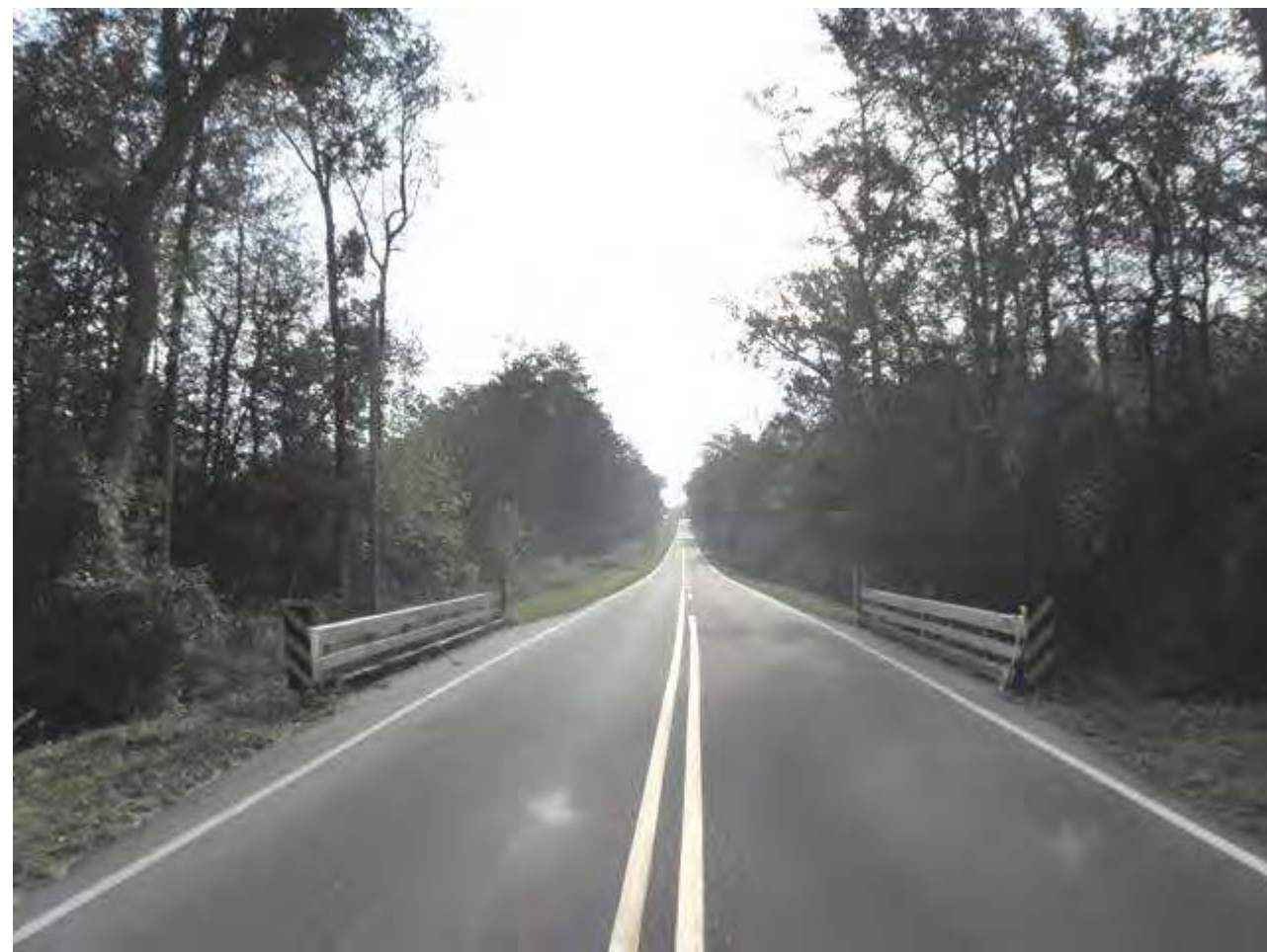
View Facing East (Upstation)
